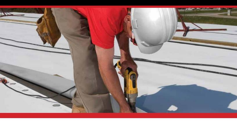
Light-colored roofs reflect UV radiation and improve a building's energy efficiency. ReflexEON TPO has the highest solar reflectivity of any TPO roofing membrane after 3 years of aging as tested by the Cool Roof Rating Council (CRRC). Its enhanced formulation provides uncompromised weatherability and durability year after year.
